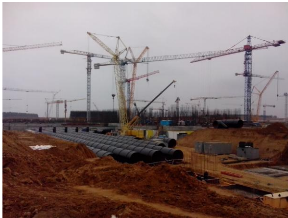
Condenser cooling pipes
