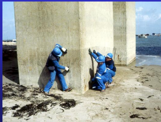
Cathodic Protection
