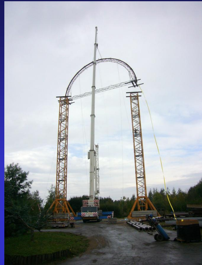
Mock up for inverted U tendons
