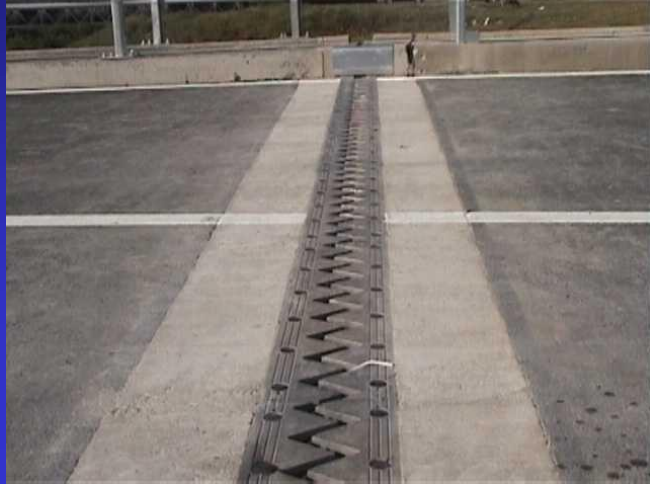
Bridges Expansion joints
