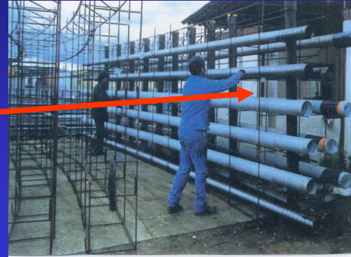
Placing of 55 T 15 ducts in prefabricated reinforcement
