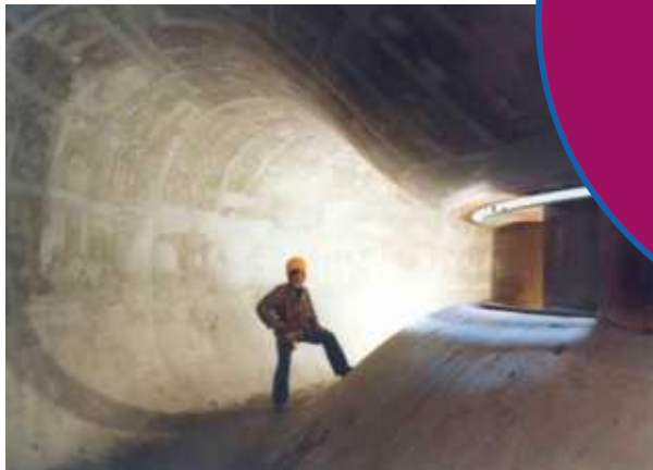
Main circulating water pump
