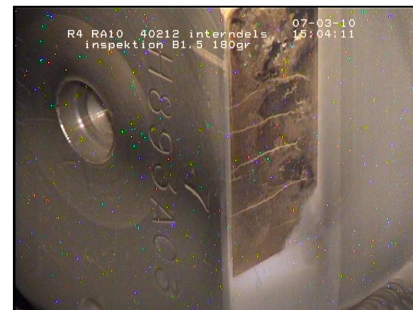
Cracks in the stellite surface
