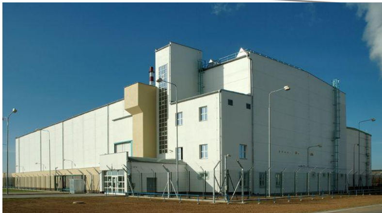
Store for burnt-out nuclear fuel, Dukovany, Czech Republic
