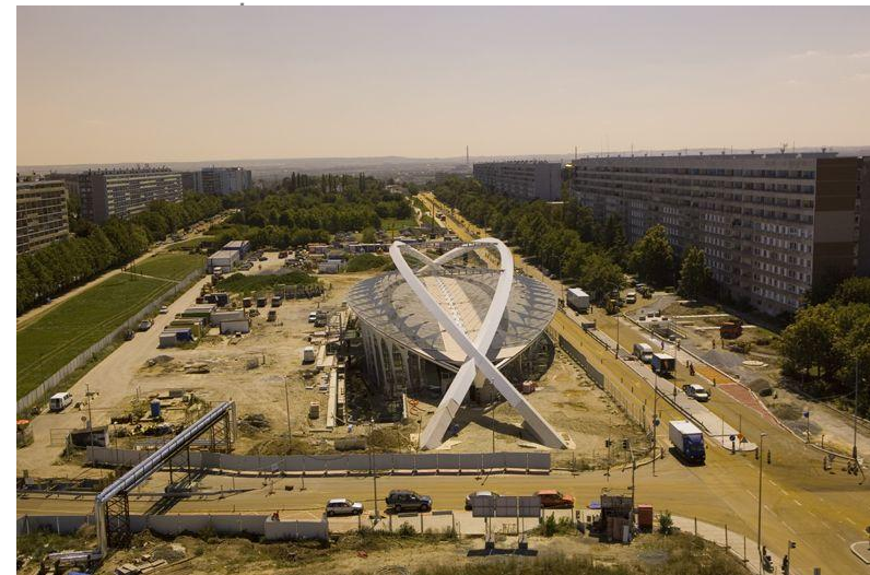
Underground IV.C2 Střížkov, Prague, Czech Republic
