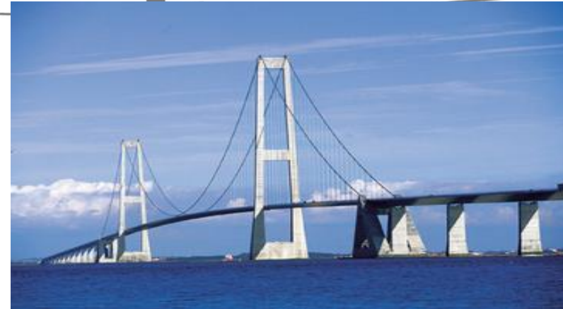
Great Belt East Bridge, Denmark
