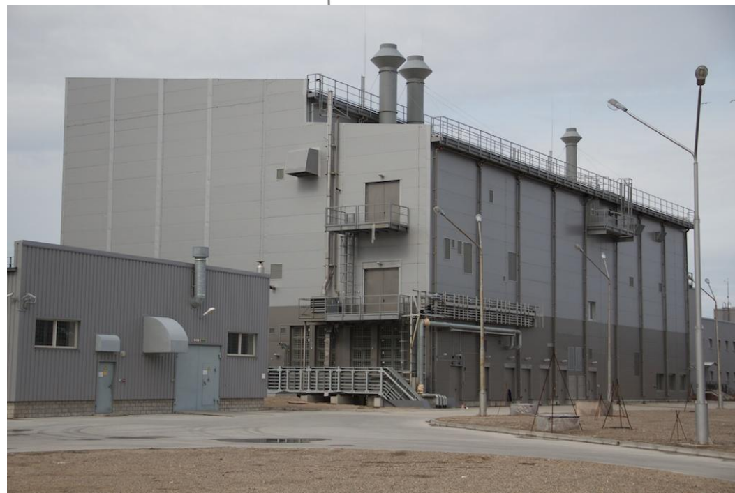
Complex for long-term storage of nuclear submarine reactors, Murmansk, Russia
