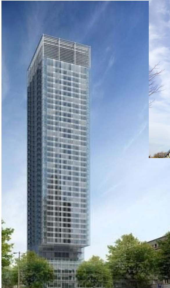
Twarda 2/4, apartments in Warsaw, Poland (under construction)
