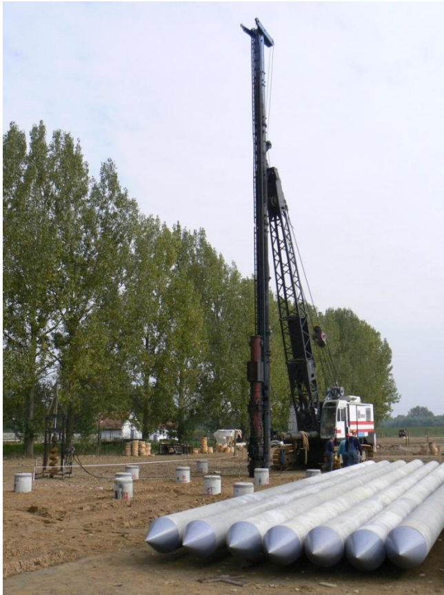
Pile – droving machine
