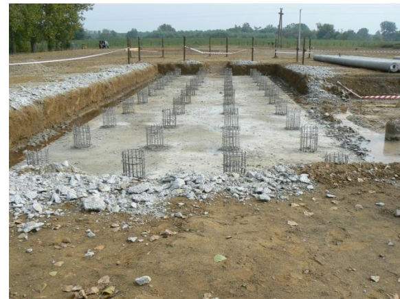
Heads of piles
